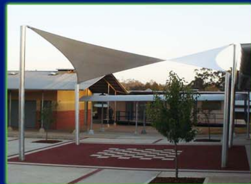
Architectural PVC Sail Macarthur Anglican School
